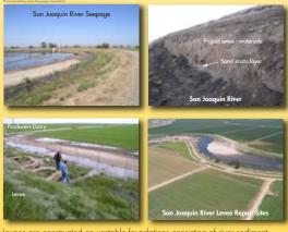
Levees are constructed on unstable foundations consisting of river sediment, mostly sand bars and sand strata. Even low flows can result in numerous sand boils and often levee failure in some reaches.
